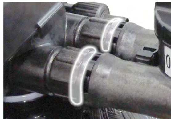
11b (Connected Properly)
